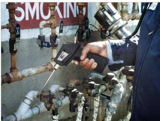
Test steam traps
